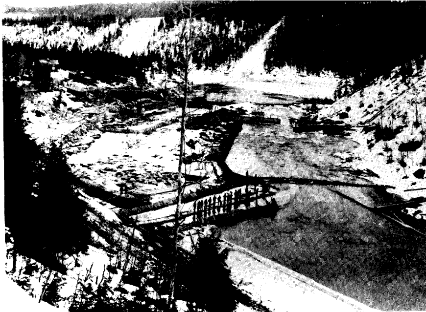
Blasting, extraction of stone and foundation work for Wiforsens powerhouse at Ljungan was carried out 1898-99. In spring of 1899 the workforce went on strike and spring floods took away dams and cranes, but in December the foundation works were completed. Photo: 1899.
