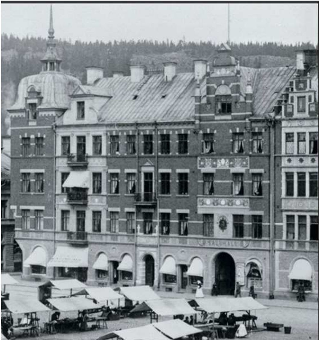
In the winter of 1895 Alfred Larsson Blomberg began excavation work for the dealer Otto Holmström's house with market place at Stora Torget. In spring the foundation was laid.
